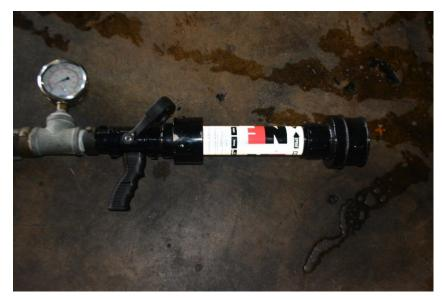
Figure 2. Handline Discharge Nozzle.
